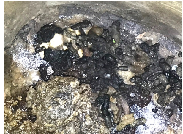
Wildlife scat in Manhole NO23-2 in 2019
