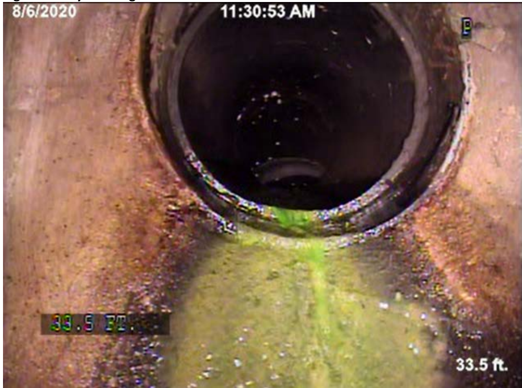
Figure 3C: Dye testing results from basement bathroom
