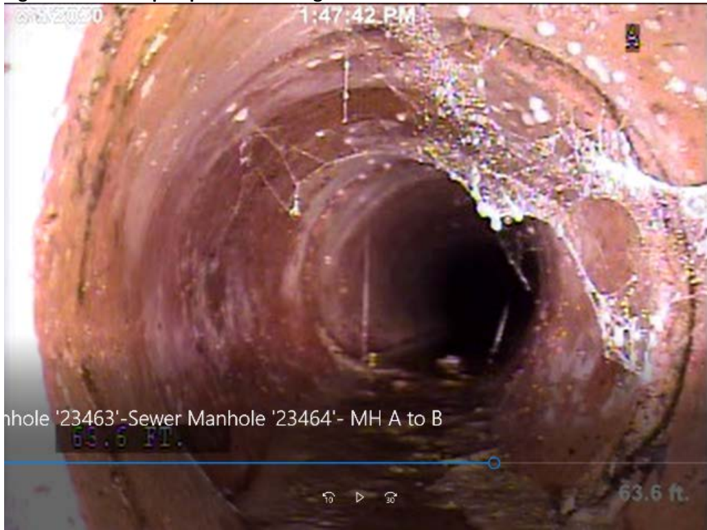
Figure 4C: Close up of possible footing drain connection – note calcium build-up in tap
