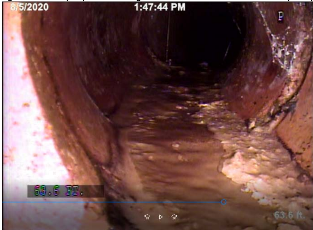
Figure 4C: Close up of possible footing drain connection – note calcium build-up in tap
